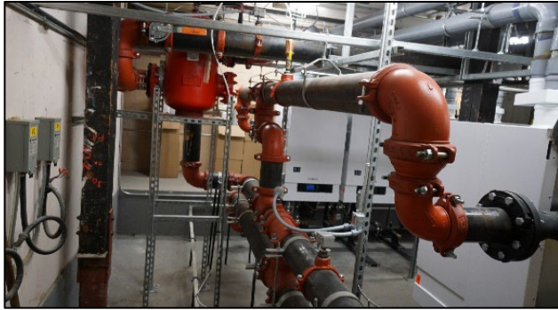
New piping for heating system at Mount Sentinel
