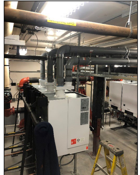
New Efficient Heat Pumps
