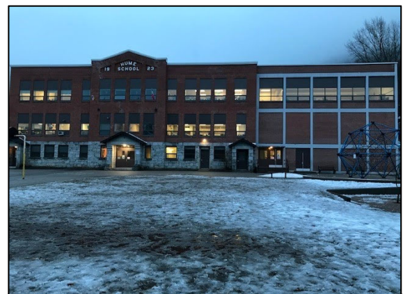
Hume Windows & Doors Replacement
