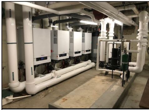
South Nelson Mechanical Upgrades
