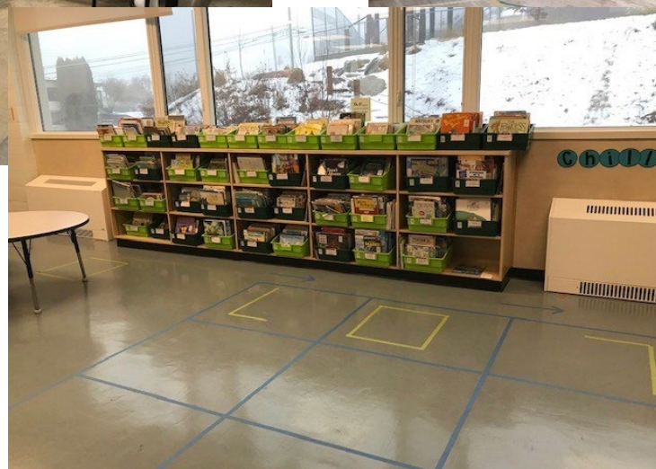
Library with new radiators & shelving
