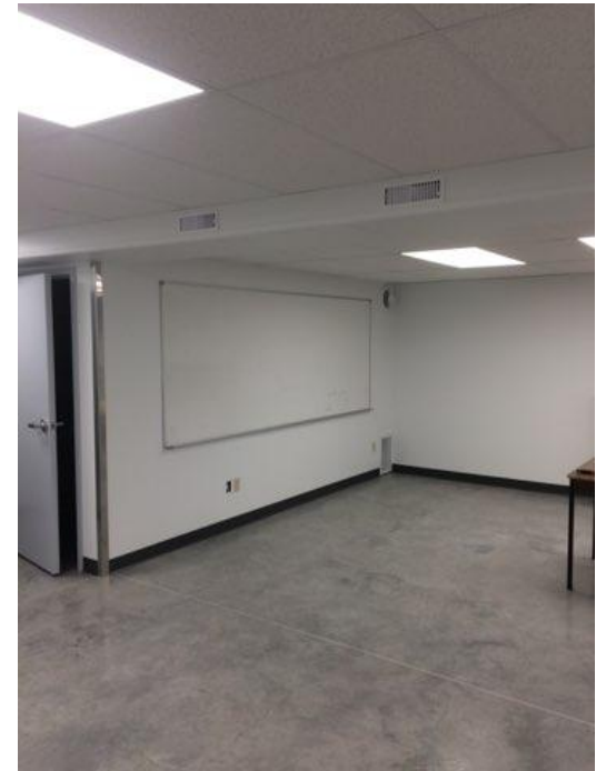
Renovated Lower Level
